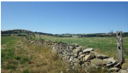
Example of stone wall that has been rehabilitated
