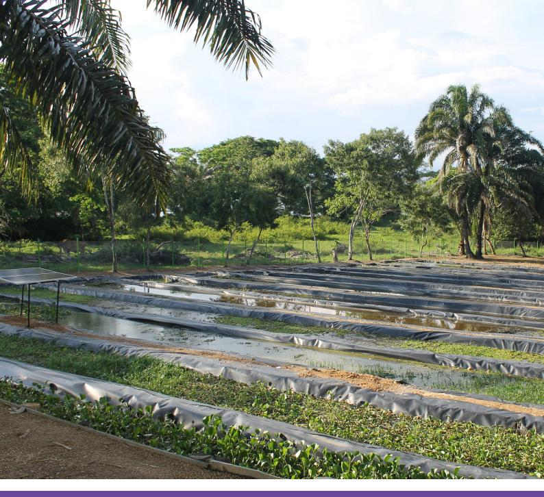
Inauguration: April 2018 Construction time: 10 months **Executor:** Fundación Humedales **Type of filter:** Horizontal surface flow constructed wetlands
