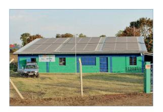
Renewable solar energy is the main energy source for the hubs. A bank of batteries is provided as backup and a generator is used in the rare instances of a lack of sunshine.
