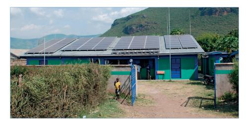
WE!Hubs are decentralized water and energy stations. Electrical energy is provided by 72 solar panels, with a performance of >220Wp each. The total installed PV capacity of >15kWp is used
