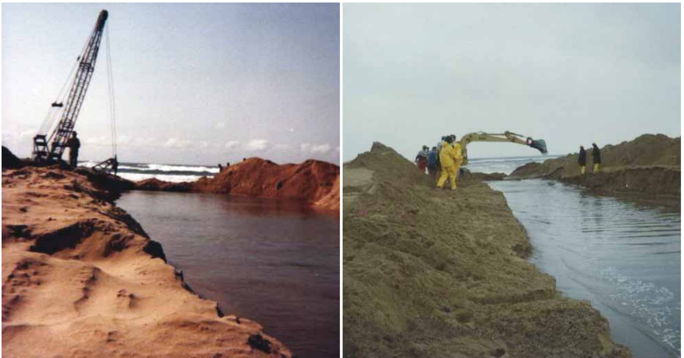
Figure 10 and 11: Artificial breaching of the Mfolozi mouth in 1979 and 1993 (photographs: N Brits)
