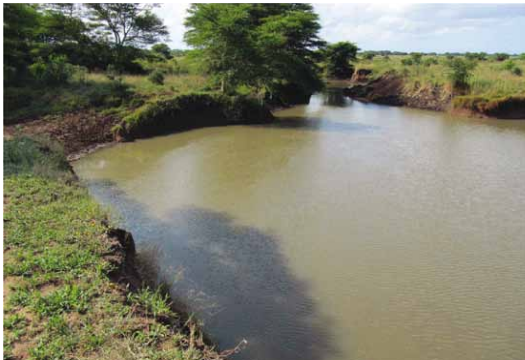
Figure 19 and 20: Erosion of the Mpempe channel caused by increased water flow as a result of the straightening of the channel to bypass the pan and bring water from the Mkhuze catchment into the lake (image and photograph courtesy of P Grundling).
