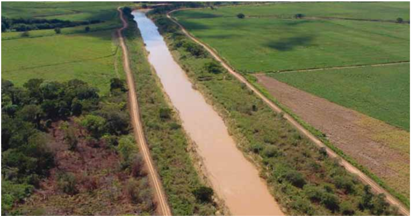
Figure 18: The canalisation of the Mfolozi river has led to an increase in the speed of the water flow. (photograph: Ezemvelo KZN Wildlife)
