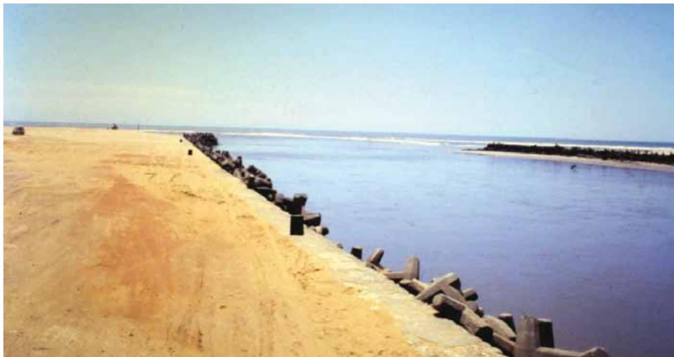
Figure 12: Lake St Lucia estuary mouth in 1983 showing the retaining walls and dolosse keeping the mouth open. (photograph: A.T. Forbes)
