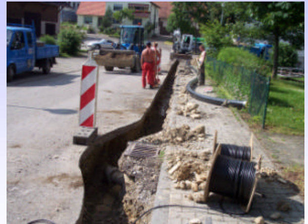
Pipe trench in Mauenheim
