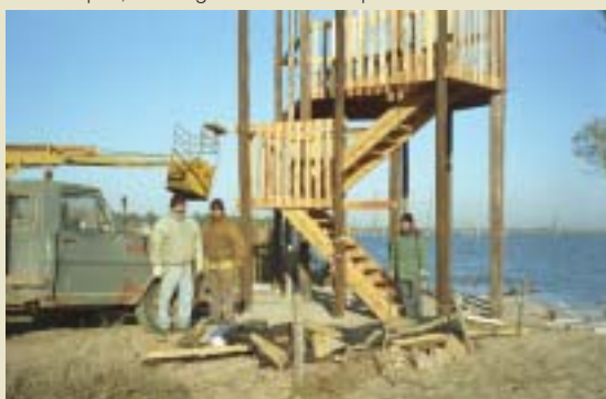
Mar Chiquita; Building the observation platforms
