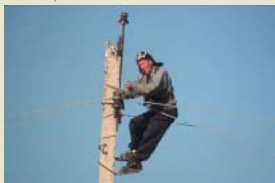
Removal of power lines
